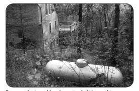
Propane is stored in a large tank. It is used to provide energy for heating, cooking, and drying clothes.
